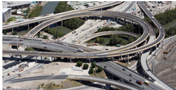
Figure 2: An example of the junction of the Tunnel, Airport Link and Inner-City Bypass in Brisbane, adopted from (ROADS AUSTRALIA, 2015)
