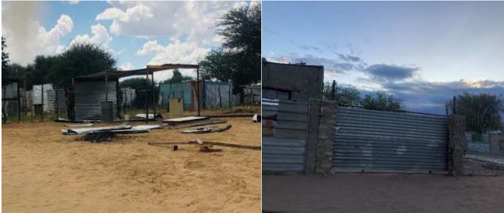
Overnight erection of new shacks and permanent structures
