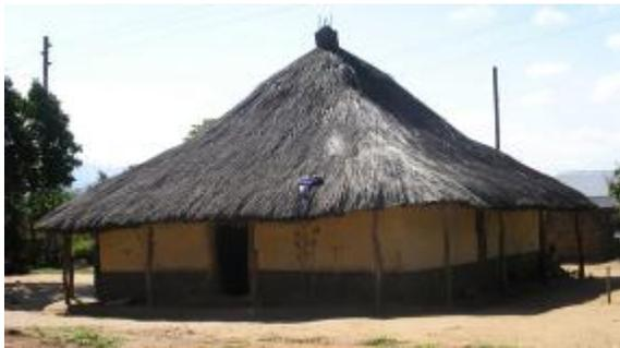
Figure 1: Typical traditional house, with raw bricks walls and thatch roof.
