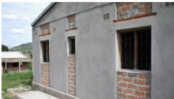
Figure 9: Informal house, with raw bricks, cement plastering walls and roofed with iron sheet.
