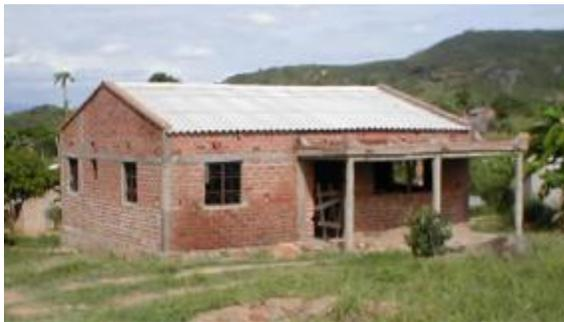
Figure 2: An improved traditional house, with raw brick walls and zinc roof.
