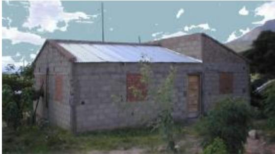
Figure 8: Informal house, with cement block walls and roofed with iron sheets.
