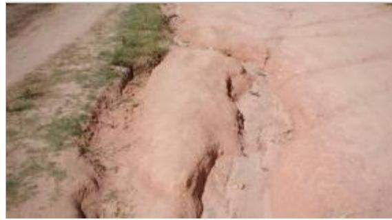
Figure 3: The erosion phenomena on the main settlement access road.
